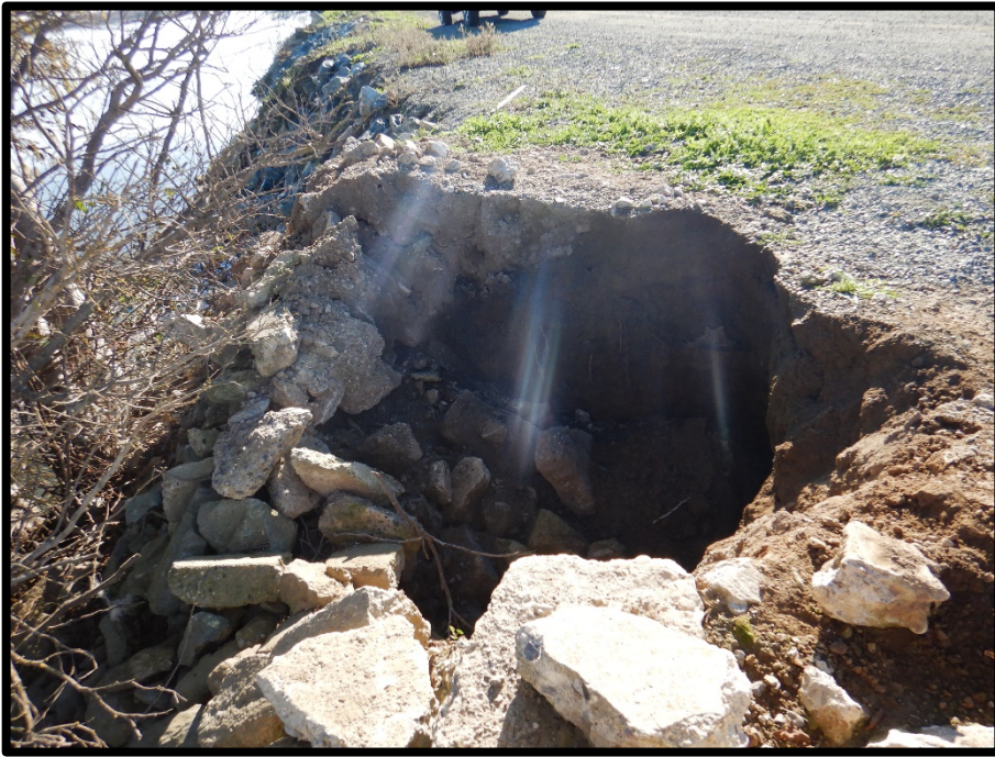
Pre-existing sinkhole on levee crown, Station 257+00. Facing south.
