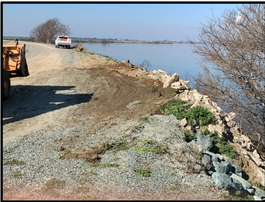
Excavated site was furnished with Class II \frac{3}{4} " AB. Facing north.
