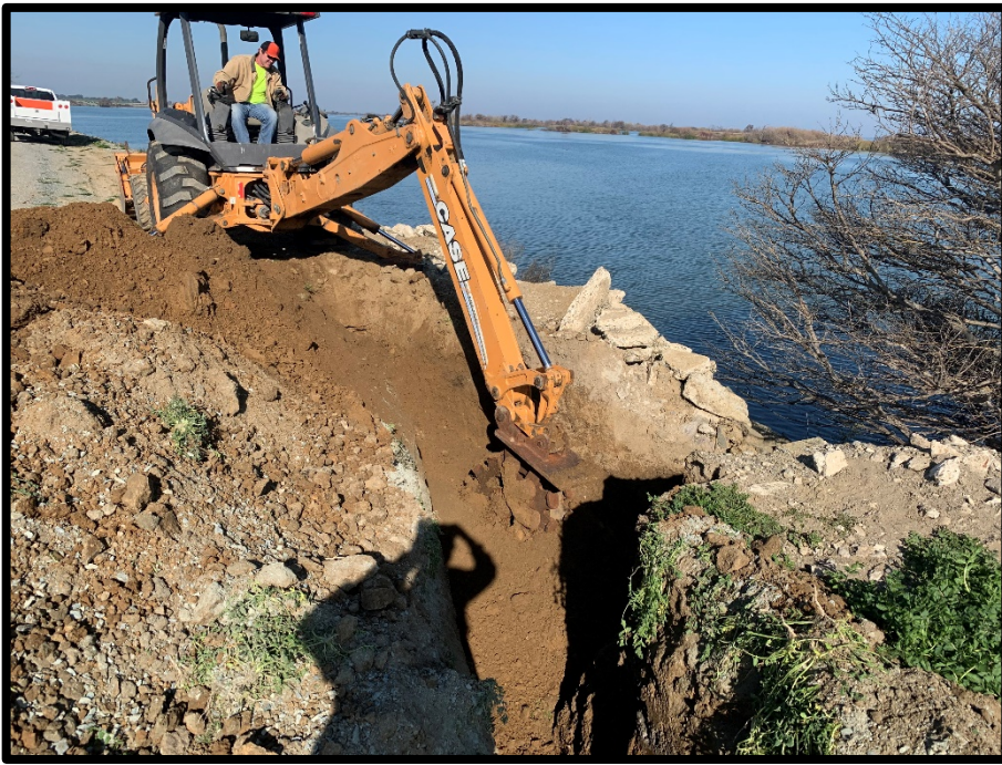
Case 580 backhoe with sheep's foot compactor attachment compacting excavated sinkhole and adjacent 25-foot exploratory trench.
