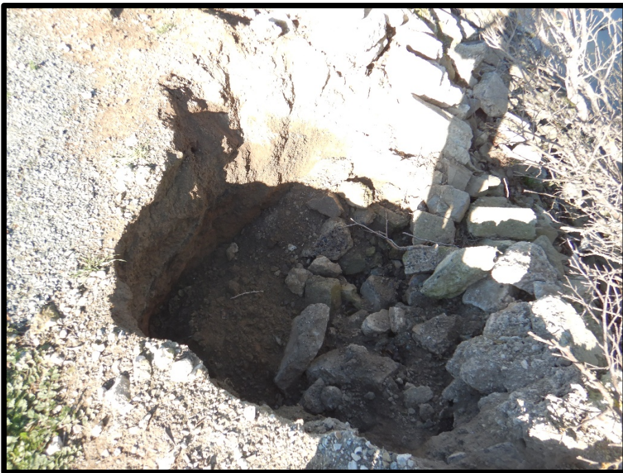
Pre-existing sinkhole on levee crown, Station 257+00. Facing north.
